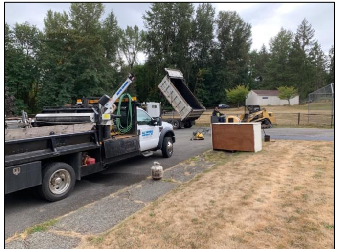
Widening the the upper-campus road
